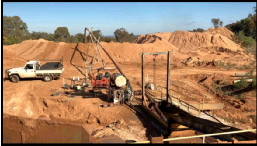
Tailings dam pump (Photo: Brian Holden)
