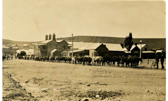
Boiler in Commissioner St, Kyloe, 1910
