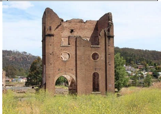
Figure 12 Lithgow Blast Furnace ("hot house")
