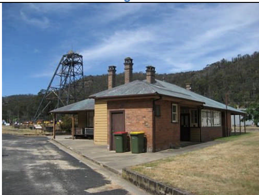
Figure 13 Lithgow State Mine Heritage Centre with head frame and outer display building.
